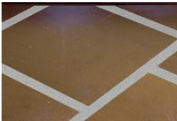
Fiber board with seams taped
