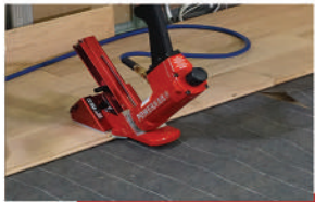
Direct Nail Down Installation
