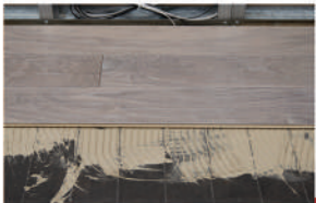
Direct Glue Down Installation
