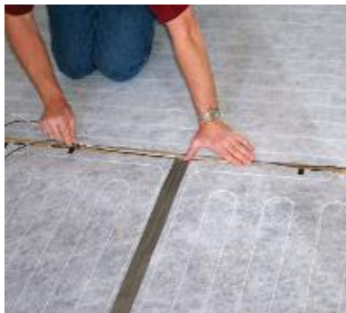
Run Lead Wires, Tape Seams
